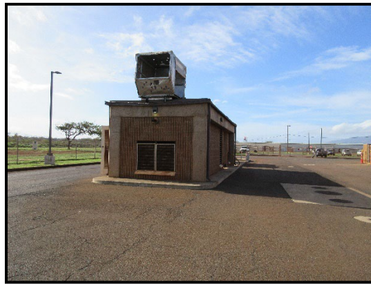
ARFF Station December 2022
